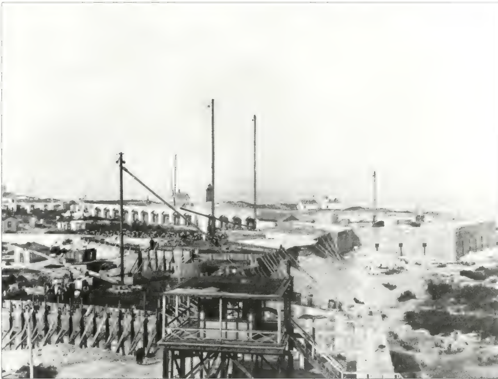
Figure 2.36. View looking northwest at construction of Nine Gun Battery, 1897. Construction began on a three-gun emplacement (center) in 1897 that would become the first component of the Nine Gun Battery. The first phase was built over the east facade of the Civil War-era granite fort whose projecting bastions can be seen in the photograph. The east facade of the fort and the new concrete battery paralleled the main shipping channel along Sandy Hook's eastern shoreline (GATE 7880).
